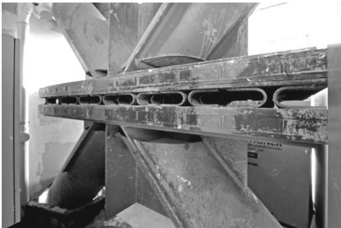
Energy dissipaters make these kinds of building structures possible, by offering a high level of security in the event of a severe earthquake or extreme winds. The dissipation of energy is allowed by special devices in the structure that reduce deformations and structural stress.
