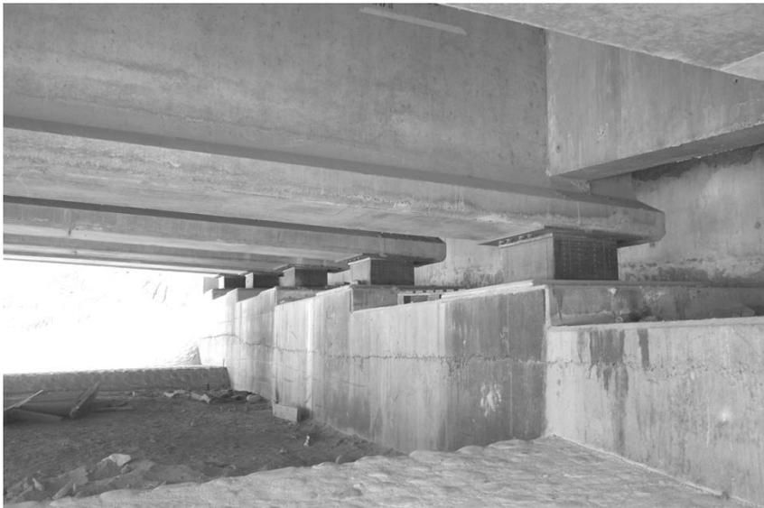
The connections between steel girders and piers, and steel girders and abutments are provided through rectangular, high-damping rubber seismic bearings. All the isolators are 300 mm high, with 204 mm of rubber, 16 reinforcing steel shims of 3 mm thick and two 25 mm steel plates at the top and bottom surfaces.
