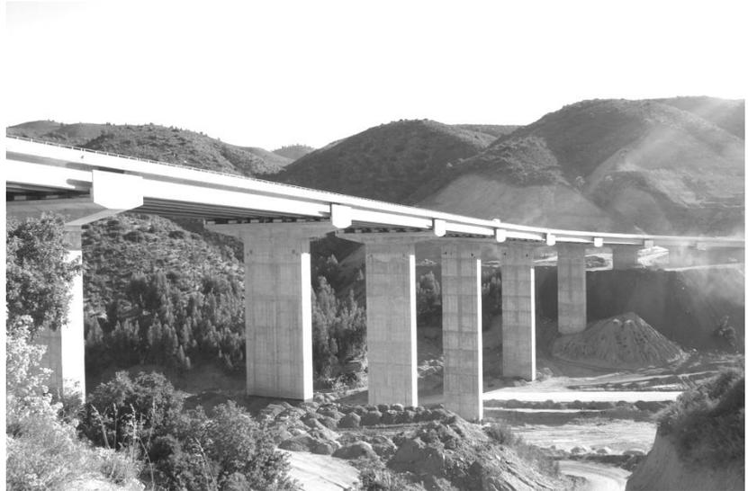
Seven piers support the girders. Pier height varies from 22 to 30 m, the tallest one located near the north abutment. A hollow-box type 2x10 m section, 0.25 m thick, is provided for all piers. Concrete cylindrical strength of 24 MPa was used in all concrete pier elements.
