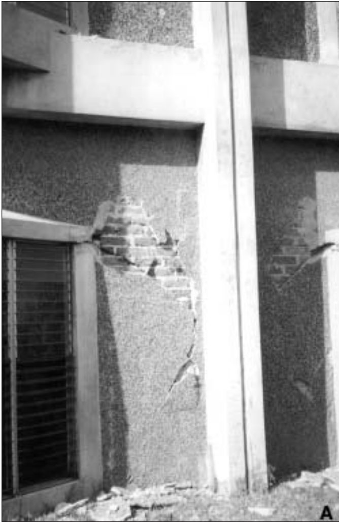
Figure 9. Damage to partition and facades due to inadequate isolation. San Rafael Hospital.
