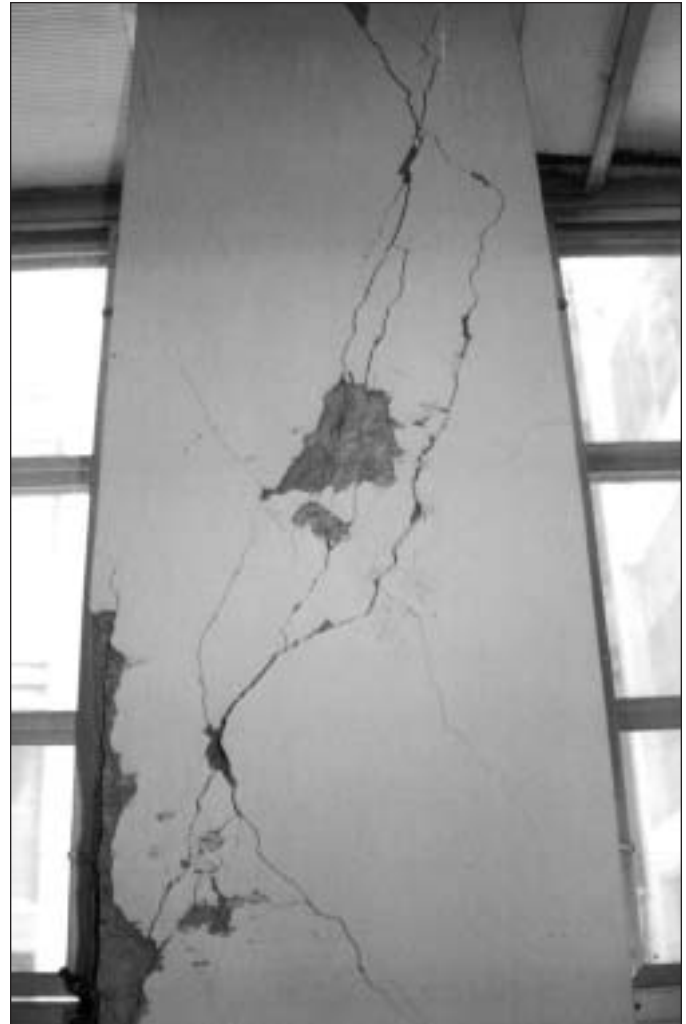
Figure 12. Shear failure in column due the presence of partial-height infilled walls. Zacatecoluca Hospital.
