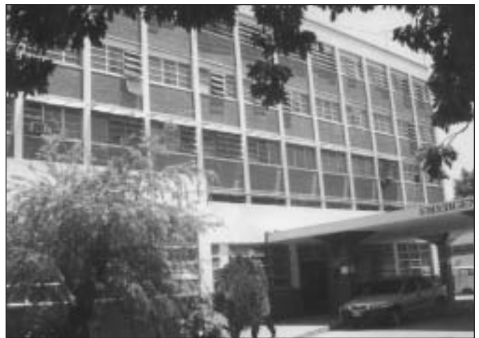
Figure 7. Typical structural system based on frame and infilled wall system.
