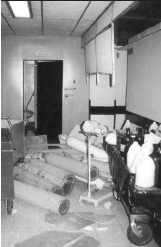
Figure 11. Medical equipment and supply damage. Surgery Building, Rosales Hospital.
