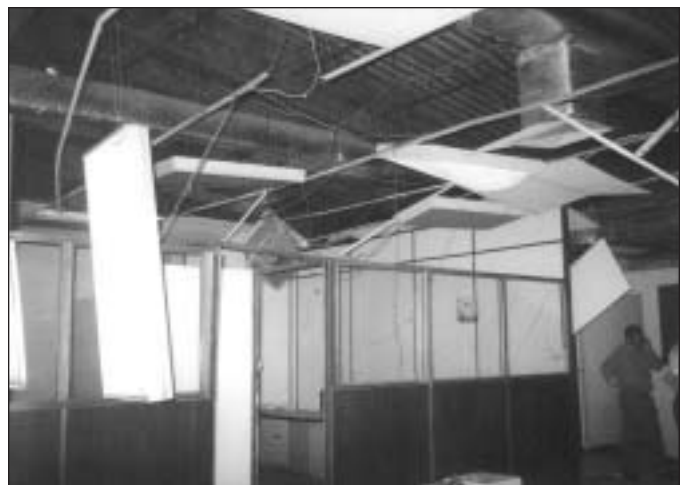
Figure 8. Damage to suspended ceiling, lighting fixtures, and air conditioning. Fertility building in Maternity Hospital.
