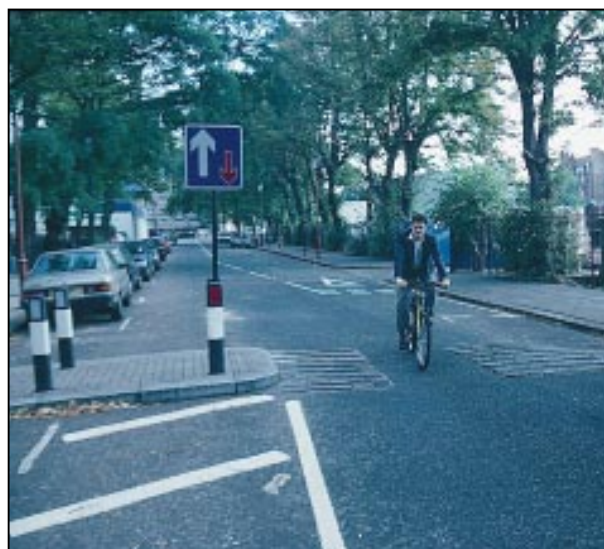
Photograph 23.3: Rumble strip with cycle-gap, Kensington. Courtesy: TRL.
