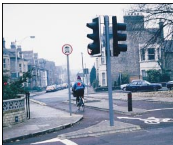
Photograph 23.8 Bypass to traffic signals and entry restriction.
