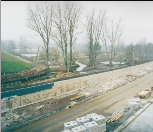
Photograph 17.8: Visual and noise barriers under construction.
