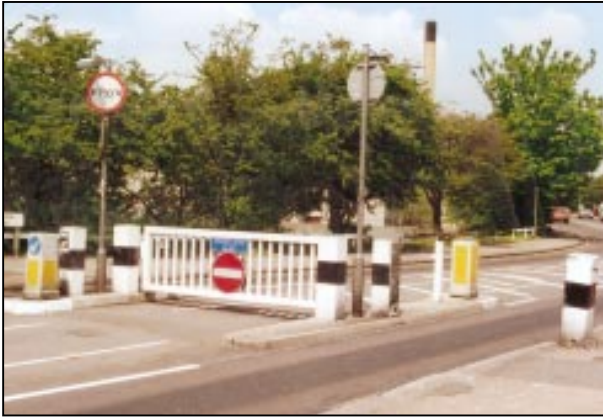
Photograph 25.3: A typical width–restriction with a gate for use by emergency vehicles.
